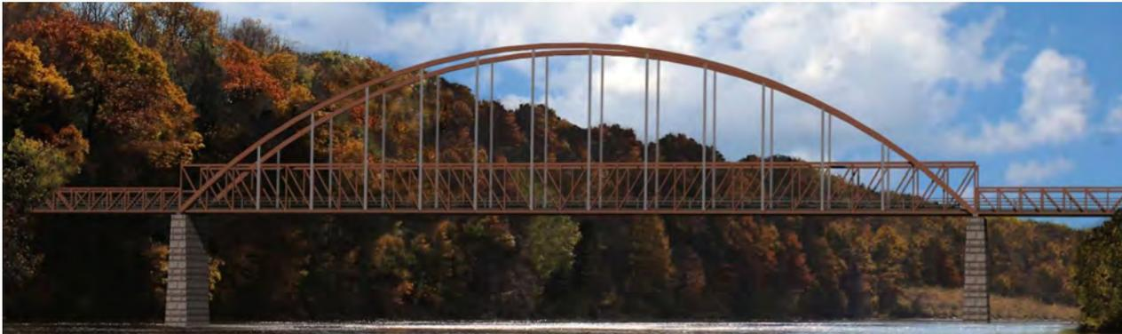
This is a tunable steel tied arch bridge. The steel horizontal deck beams are fastened to the ends of the steel arches, tying them together so that they can't spread - therefore no horizontal forces on the piers. Tunable means the tensions in the vertical cables can be optimized for dead/live loads. Community input was for a cleaner, one-height railing. *massDOT* says it will consider this.
