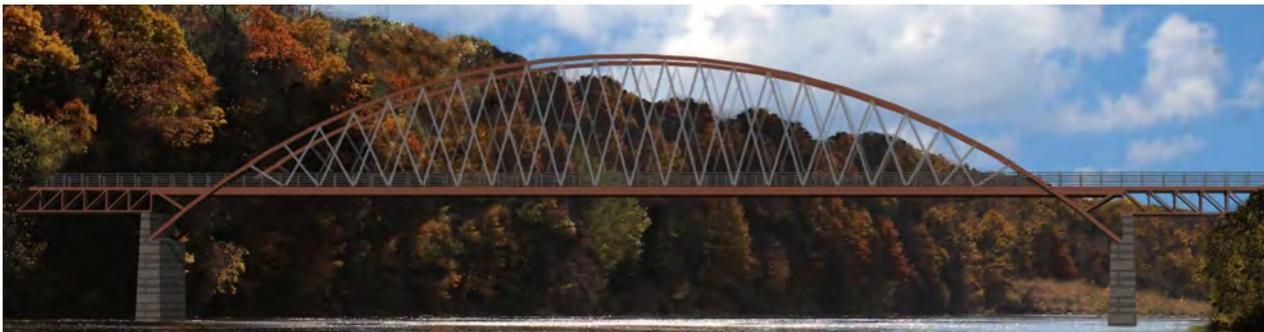
Similar to the tied arch design above, but having a cleaner railing system. The non-vertical cables are more reminiscent of the current Schell than the vertical cables; community input was mixed on vertical vs non-vertical cables. *massDOT* will consider a version with five pairs of vertical cables.
